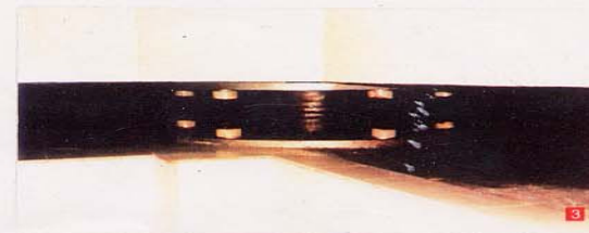
隔震垫节点大样 Detail of base isolation with Rubber Bearings made in Vibro-Tech
