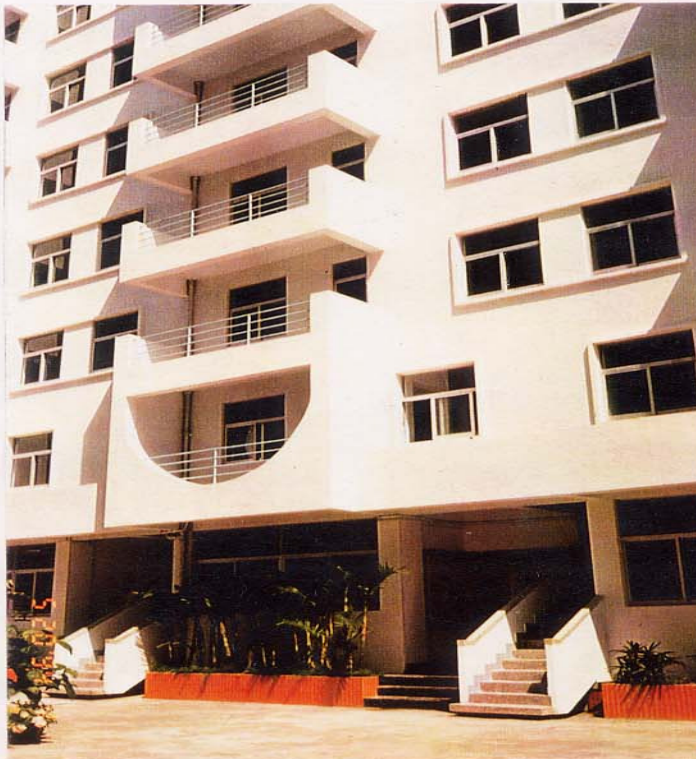
汕头市陵海大路住宅楼 Eight stories house building with base isolation in Shantou, China
