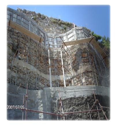
By Shotcrete with steel Mesh reinforcement supported on the nails
